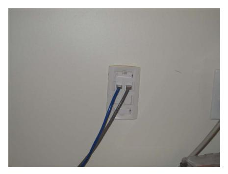
More complex: Connect device to your modem with long ethernet cabling, using drill, cabling tools, and faceplate w/terminals. \$\$->\$\$\$ (outsource)
